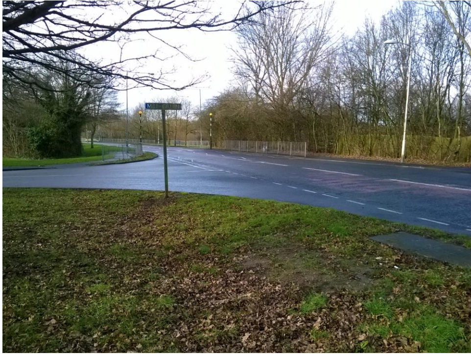
View looking west across junction with Mill Green
